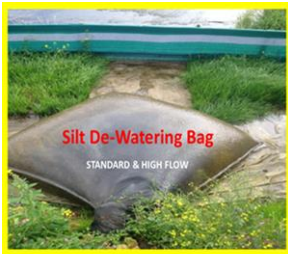
Figure 7-16 Example of silt dewatering bags
