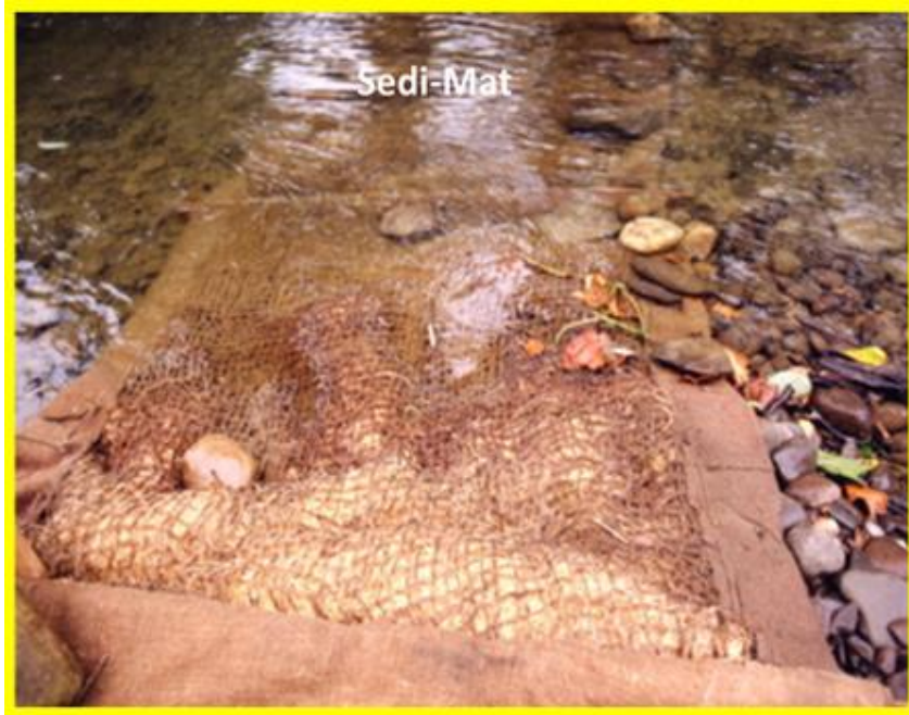
Figure 7-21 Example of a Sedi-Mat
