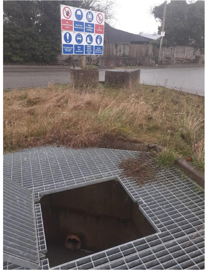
Figure 5-3 Existing stormwater tank
