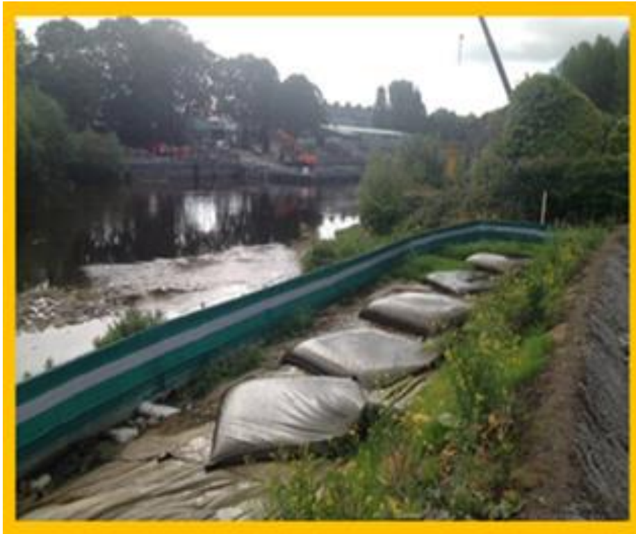
Figure 7-15 Example of silt dewatering bags
