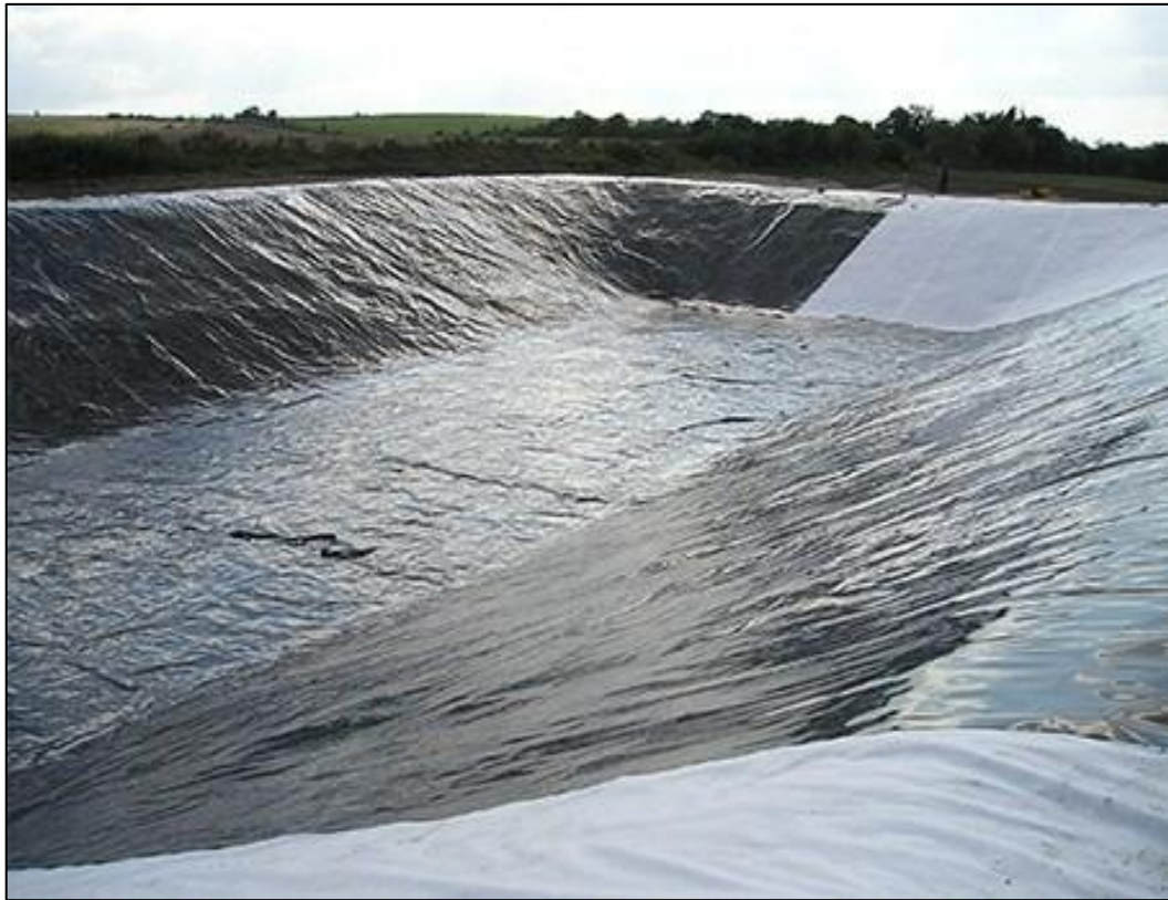
Figure 7-8 Membrane Lined Ponds
