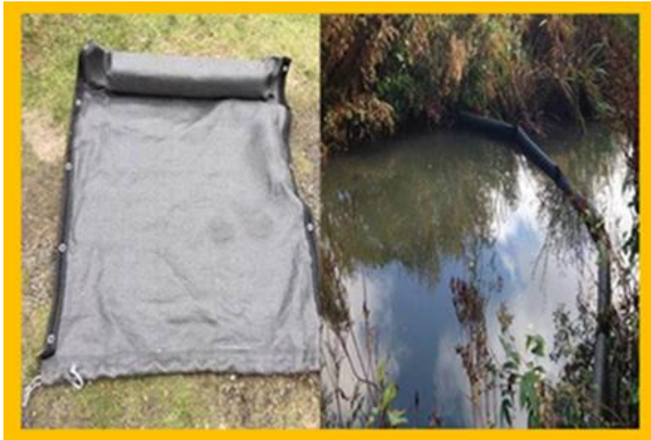
Figure 7-18 Example of a Silt Curtain
