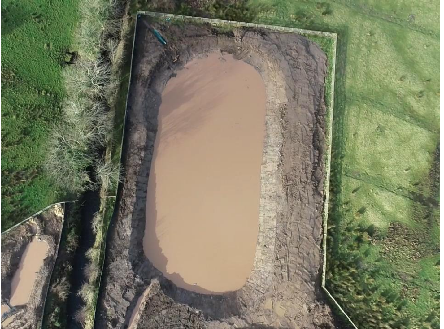
Figure 7-23 Example of a Settlement Pond
