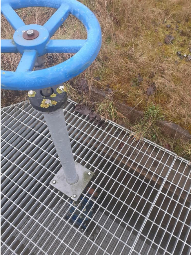
Figure 5-2 Existing stormwater tank
